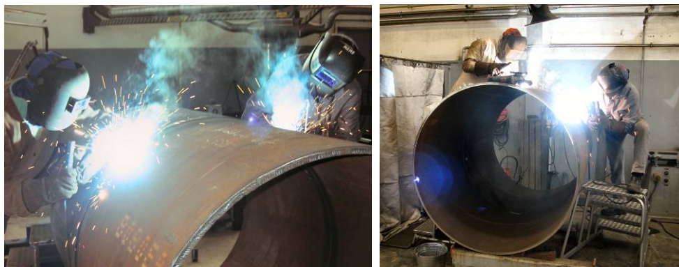
Figure 15 - Weldability assessment of X80 bend segments (SMAW)
