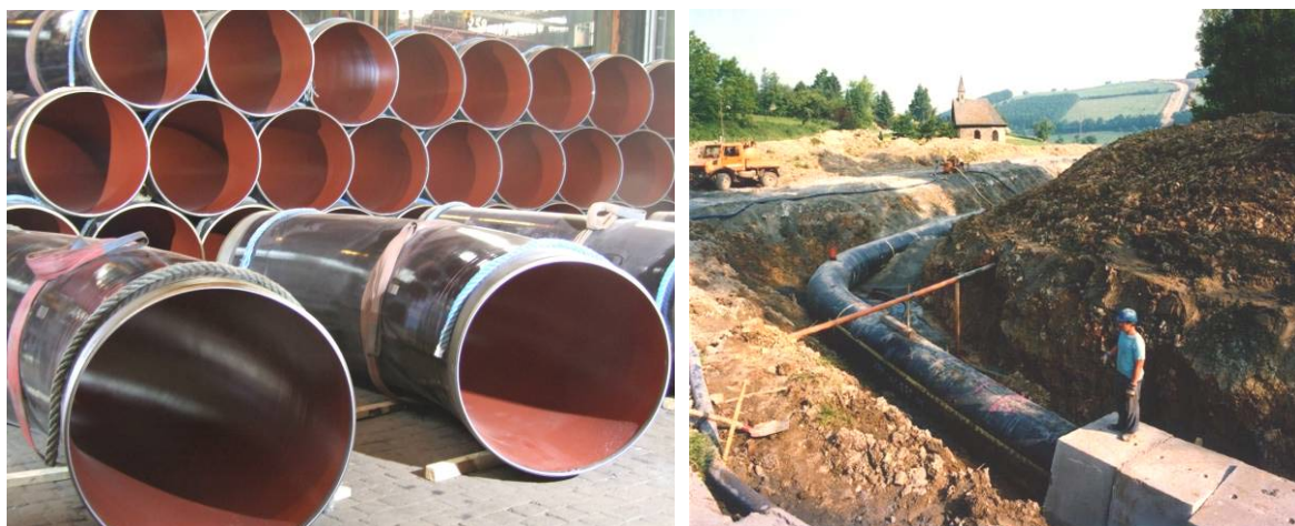
Figure 1 - X80 induction bends ready for shipment and bend in field connection
