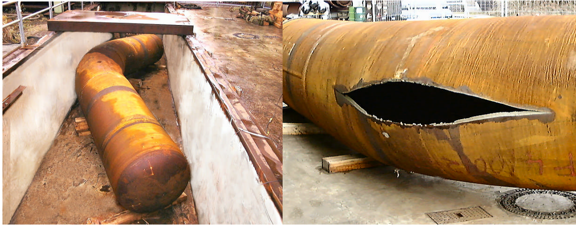
Fig. 15: Set up of full scale burst test on a high strength 48" bend at SZMF
